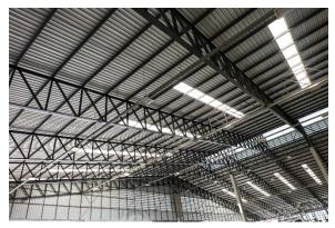
A roof system includes a roof structure and multiple layers of materials above it. The roof structure usually includes some type of deck spanning a network of load-bearing structural joists and beams. These load-bearing roof elements are less likely to be replaced unless a catastrophic failure occurs such as from a tornado or fire or long-term neglect of the roof cover. Our analysis will focus on the components above the load-bearing structural elements.
